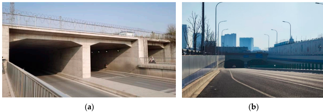
Figure 1. Tunnel photos: (a) The Luhua Road Tunnel in Beijing. (b) The Tongzhou Beiguan Tunnel in Beijing.
