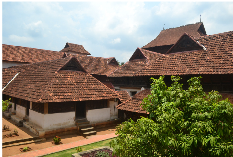
Figure 11. Gable roofs and wooden ceiling works are the prime features of Kerala's architectural style.
