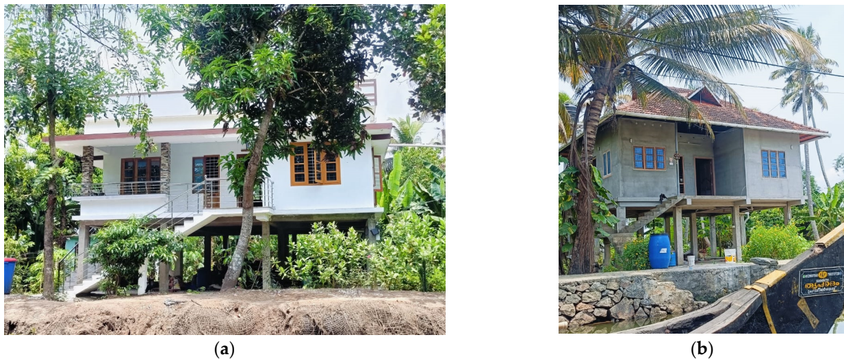
Figure 13. (a,b) Photographs of elevated houses built on concrete stilts in the Kuttanad region.
