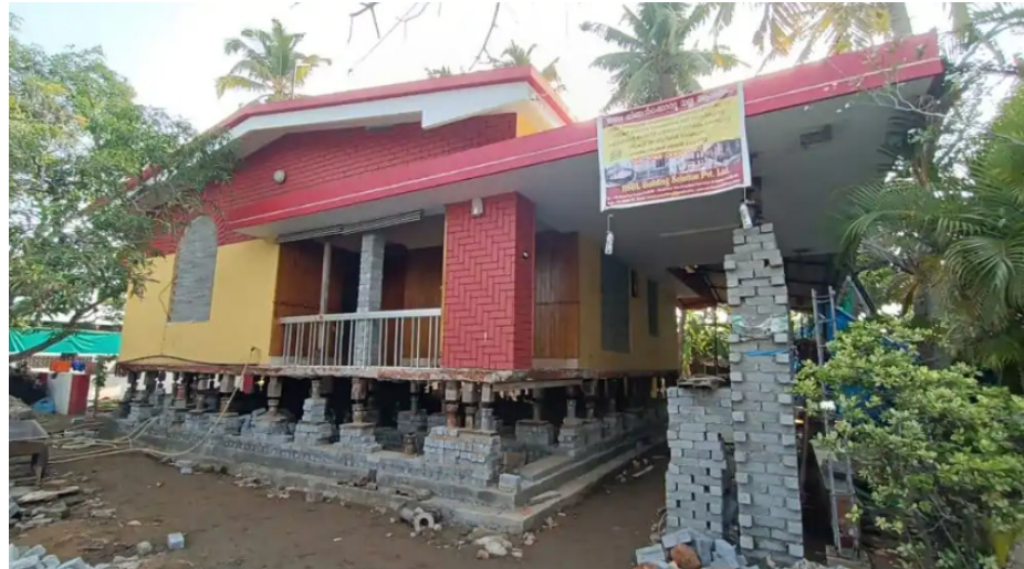
Figure 14. A house in Kuttanad using hydraulic jacks [79].
