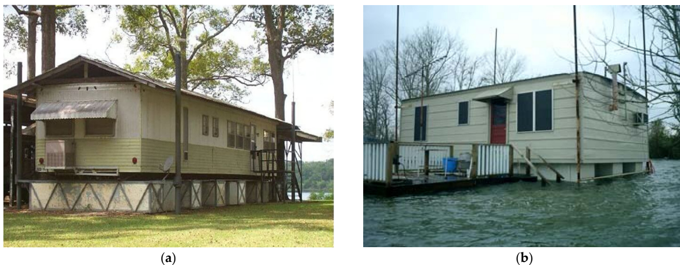
Figure 3. (a) Amphibious house with Styrofoam foundation under normal dry conditions. (b) Amphibious house floating with flooding level [34].
