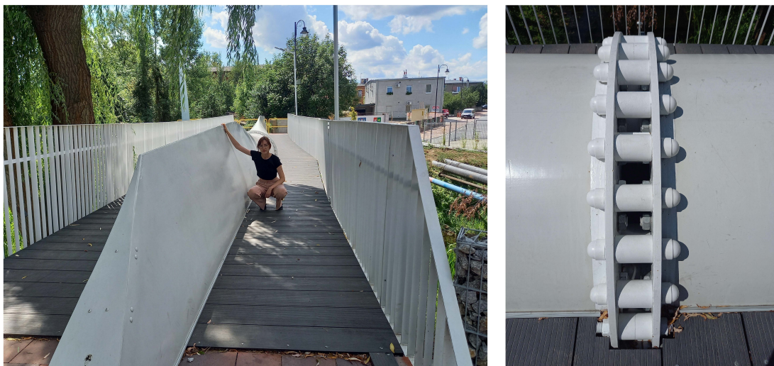
Figure 3. Footbridge in Szprotawa: flanges connecting two wind blades.
