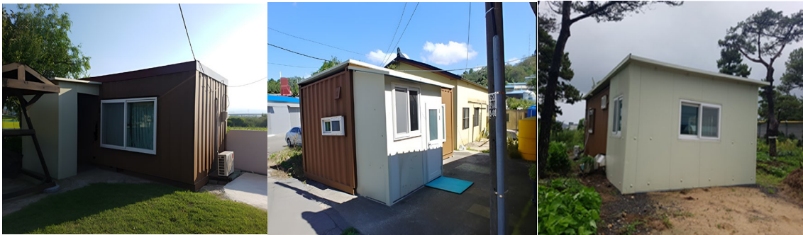
Figure 4. The case of additional space construction to prefabricated temporary housing.
