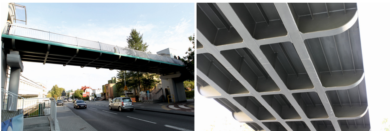
Figure 1. Side and bottom view of the footbridge in Gdynia city.
