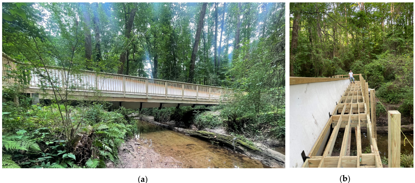
Figure 1. BladeBridge in Atlanta, Georgia, USA (2025). (a) Side view over the creek. (b) Deck sub-structure prior to deck planks being installed [18].
