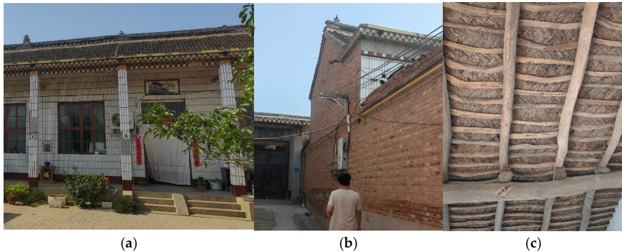
Figure 5. Figures (a–c) illustrate the pitched roof styles, external roof materials (grey tiles), and internal roof materials (wooden structures and reed mats) of vernacular dwellings in the sample villages.
