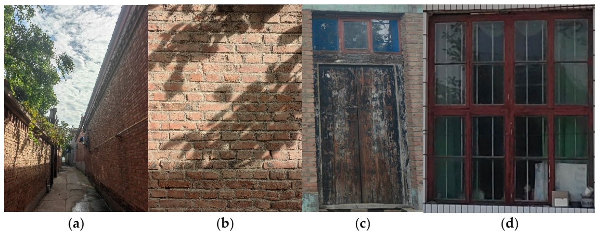
Figure 4. Figures (a–d) present the exterior wall materials, specifically 37 cm red bricks, as well as the door and window materials, which consist of wood and single-pane glass, used in the vernacular dwellings of the sample villages studied.
