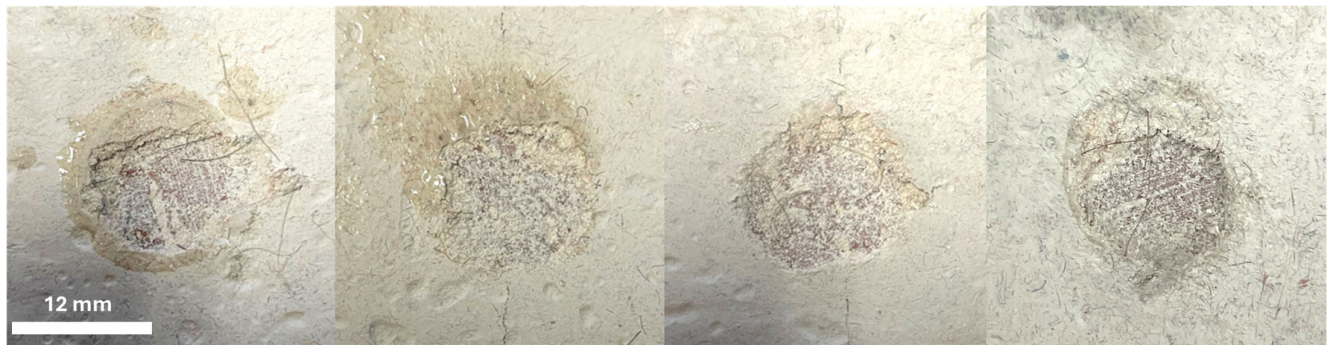
Figure 10. Dolly imprints (diameter 12 mm) showing interface failure after pull-off test on clay brick substrate.
