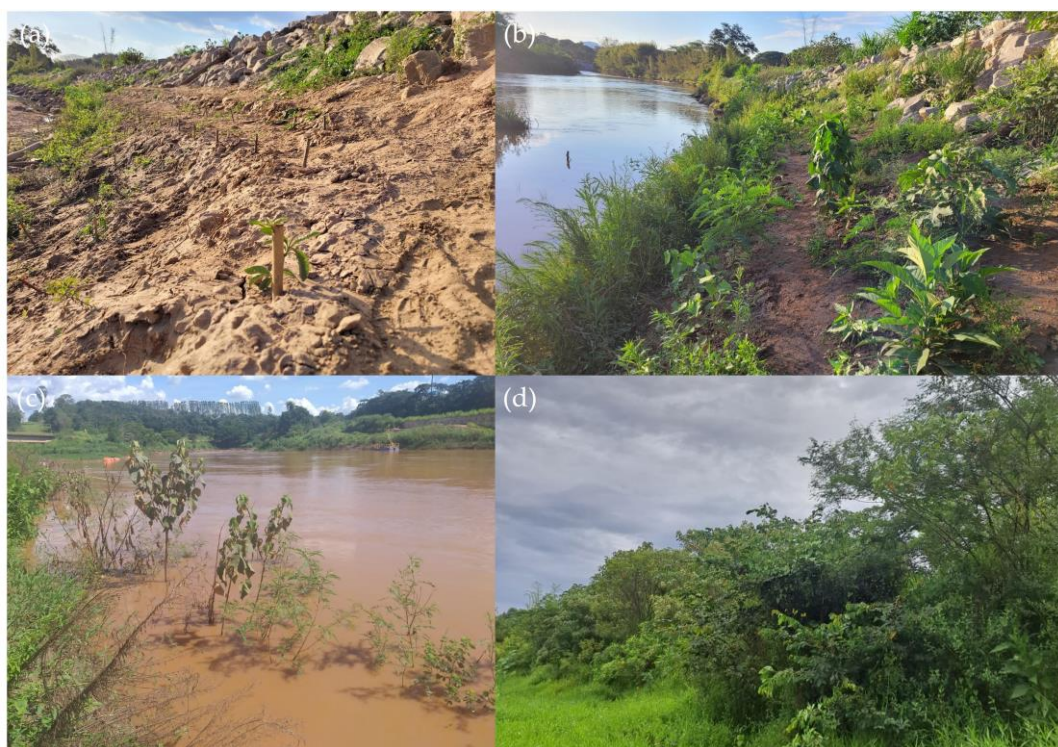
Figure 6. Temporal evolution of a soil and water bioengineering intervention using live cuttings along the Paraopeba River, Brazil. (a) Immediately after planting, showing freshly installed cuttings on the riprap slope; (b) early establishment phase, approximately three months after planting, with initial shoot development and partial vegetation cover; (c) flood event during the establishment phase, illustrating plant exposure to inundation and fluvial disturbance; (d) advanced post-establishment phase, showing dense vegetation cover and structural integration of planted and spontaneously recruited species on the riverbank.
