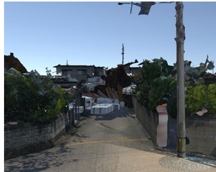
Figure 12. Street-level view of evacuation-route obstruction caused by collapse-induced debris.
