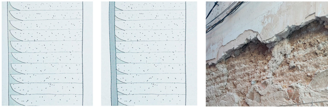
Figure 6. Replacement of the lime crust with a gypsum coating.
