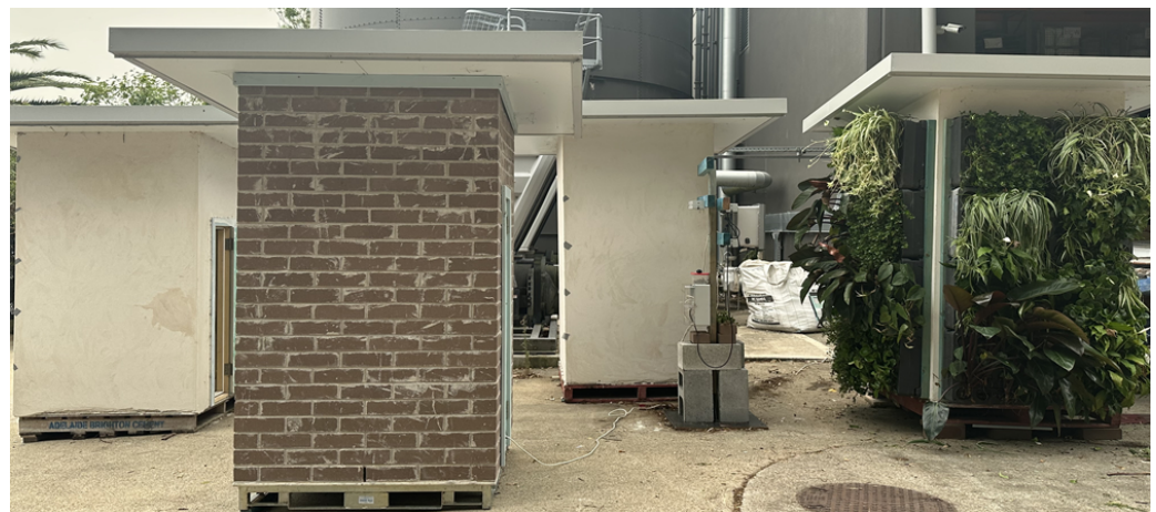
Figure 1. Test structures located within the controlled research facility (Botany, NSW, Australia). From left to right: cast in place (CIP), brick, prefabricated and prefabricated with greenwall (GW).
