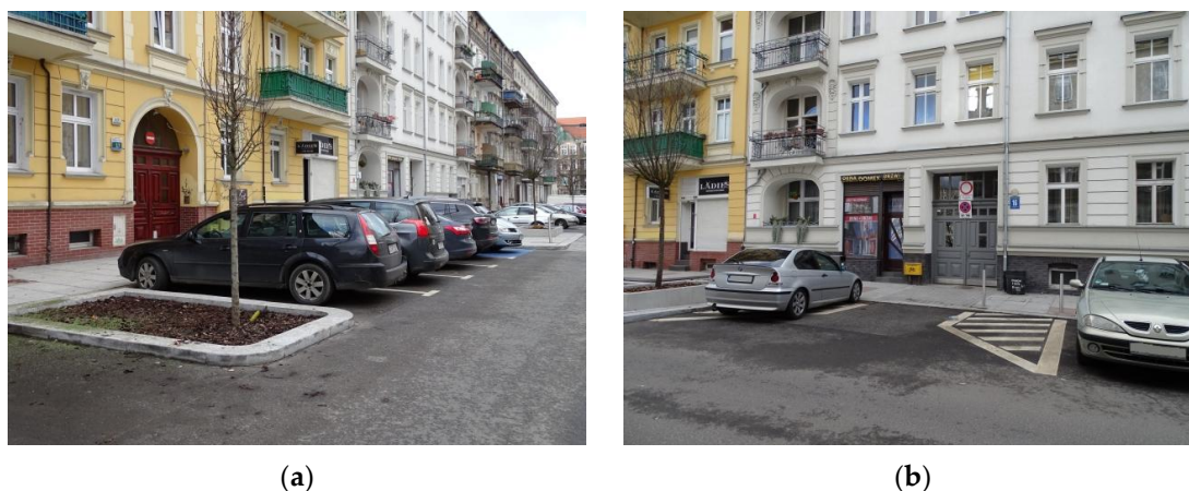
Figure 29. Examples from field observations: (a) side island constructed within a parking lane; (b) unauthorised parking on a hatched area near an access to an internal courtyard. Source: photos by the authors.
