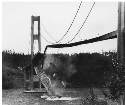
Figure 1. The Tacoma Narrows Bridge collapse.
