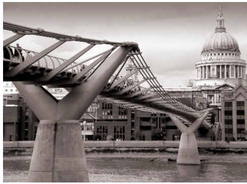
Figure 2. London's Millennium footbridge.
