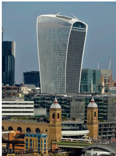
Figure 4. 20 Fenchurch Street, London.
