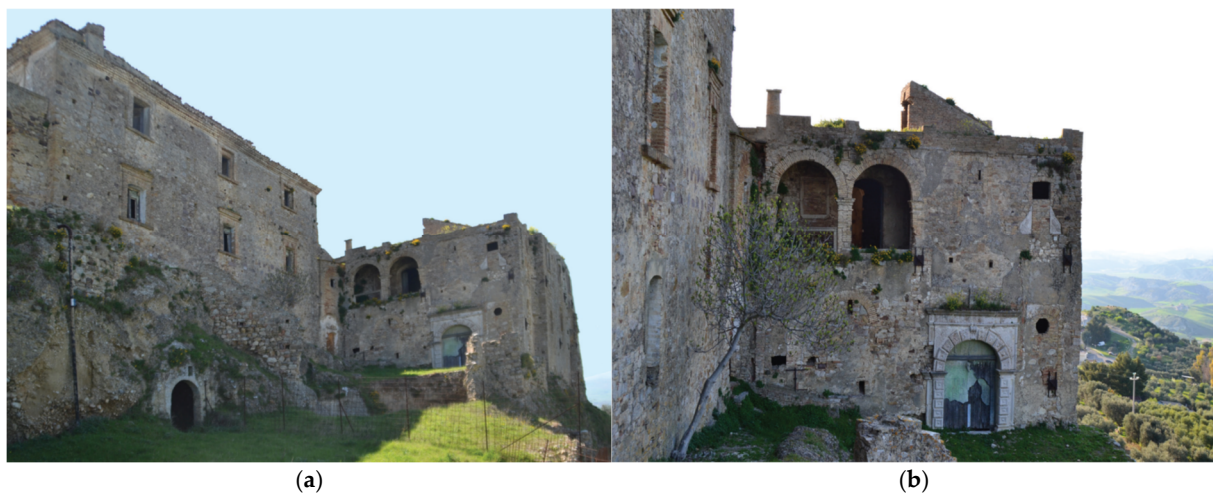
Figure 2. (a,b) View of Palazzo Carbone-Rigirone from Via Alfieri and east elevation of Palazzo Rigirone with detail of the loggia.
