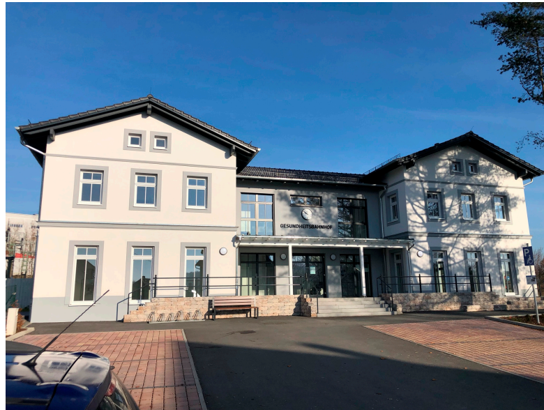
Figure 5. Doctor's office in former station building in Nöbdenitz (Arvid Krüger).
