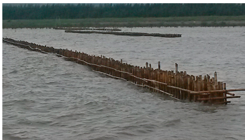
Figure 14. Bamboo with reed filling as temporary protection for mangrove planting in Vietnam (picture by author).
