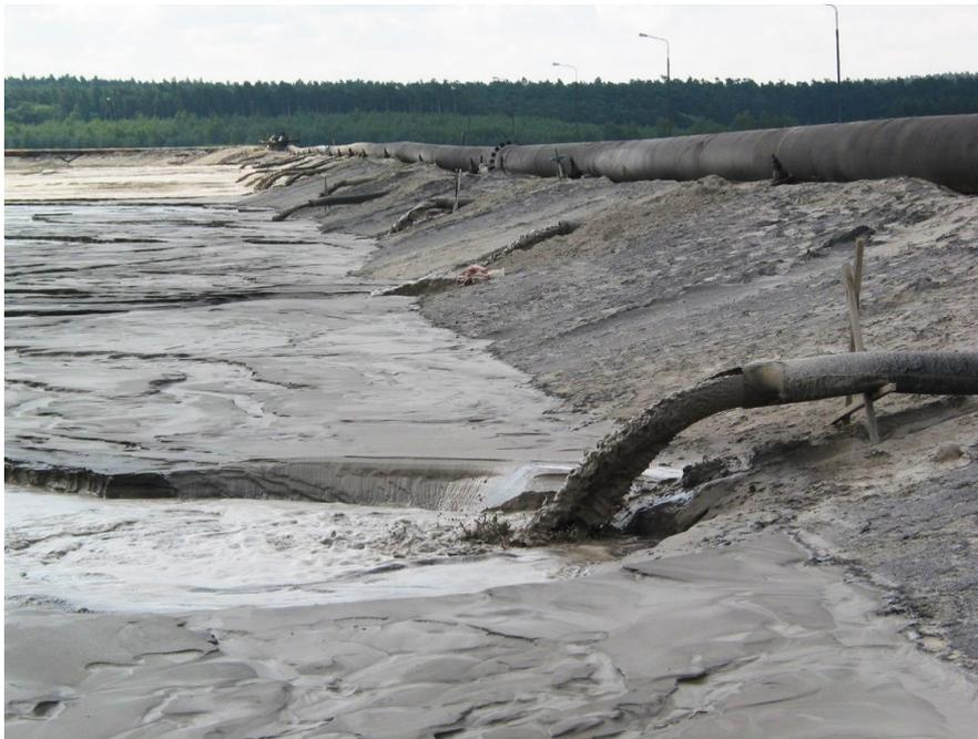
**Figure 2.** Waste spigotted onto the facility’s beach [13].
