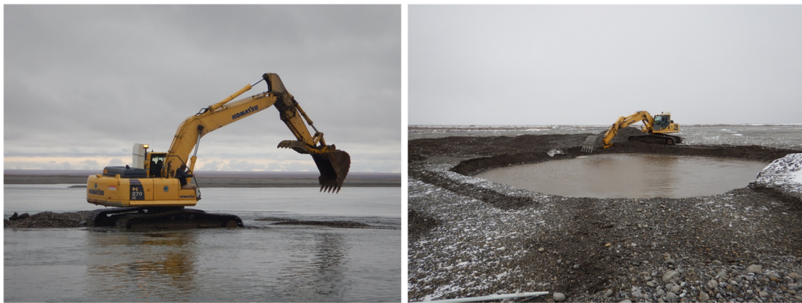
Figure 2. Field excavation of a wet pit (left) and a dry pit (right).
