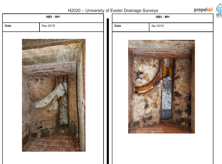
Figure 6. Photograph of Manhole HB 1 from lift and look surveys in December 2018 and April 2019. The image on the left-hand side shows a blockage in the chamber caused by a build-up of rag.
