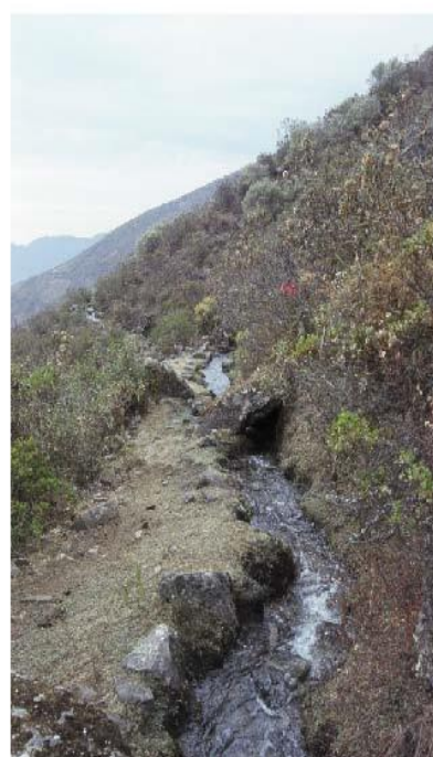
Photo right: Detail of Chorrillos-Pukio Canal flowing west towards Pukio. Note that canal has a stone-lining
