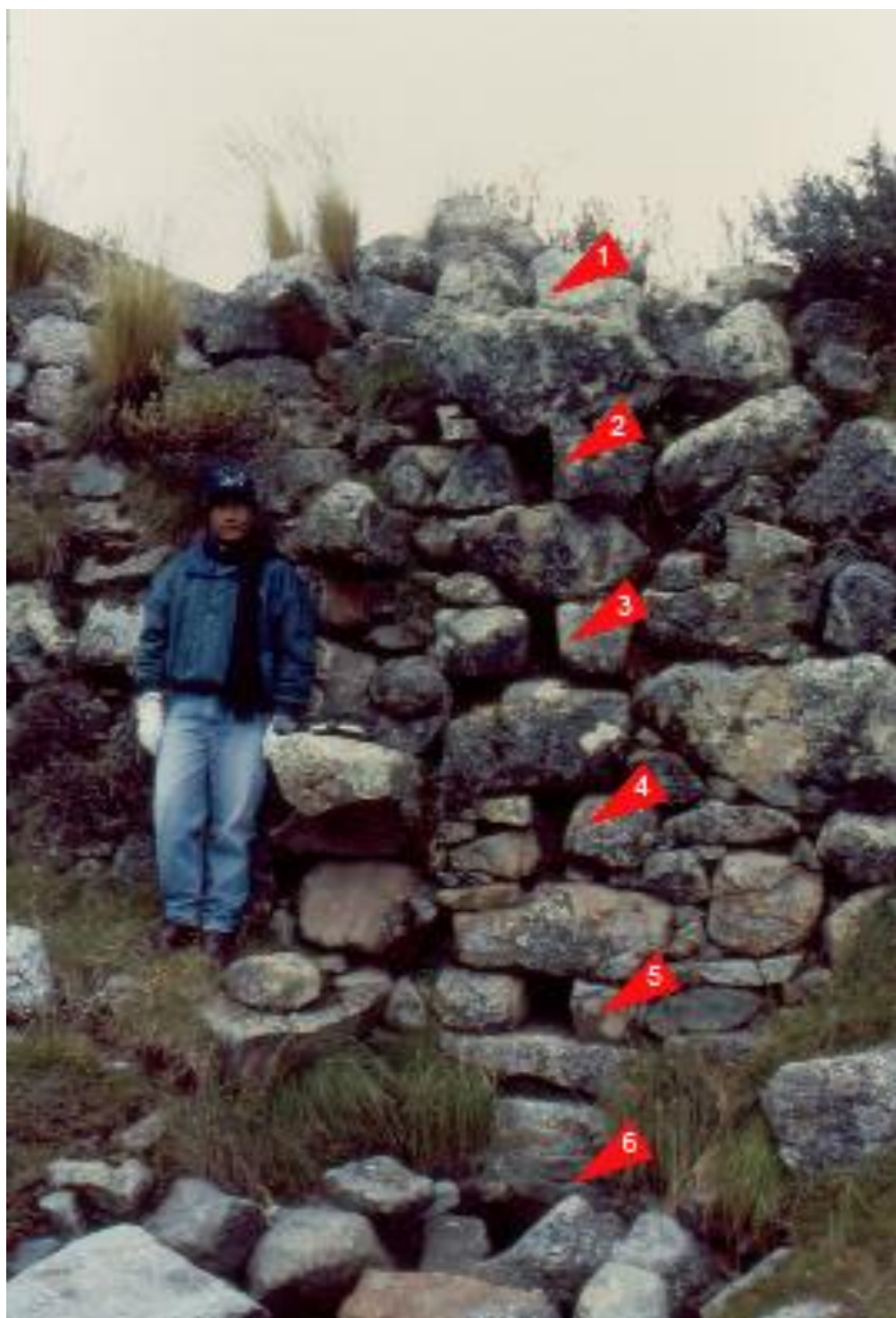
Figure 7. External face of Ricococha Baja [Ra 1] showing six sluices.
