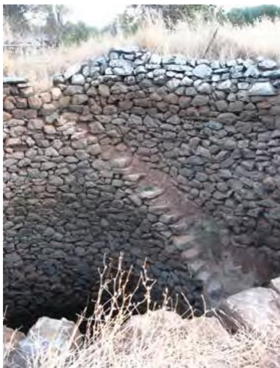
Figure 14. A cistern near Neapolis in eastern Crete which is still in use (photo: A. N. Angelakis) [82].
