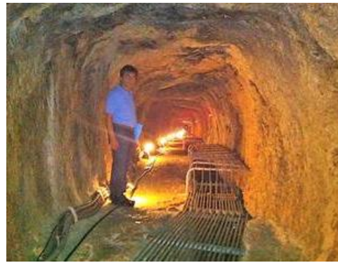
Figure 5. A view of the Eupalinos tunnel with the aqueduct channel on the right-hand side of the picture (with permission of K. Voudouris).
