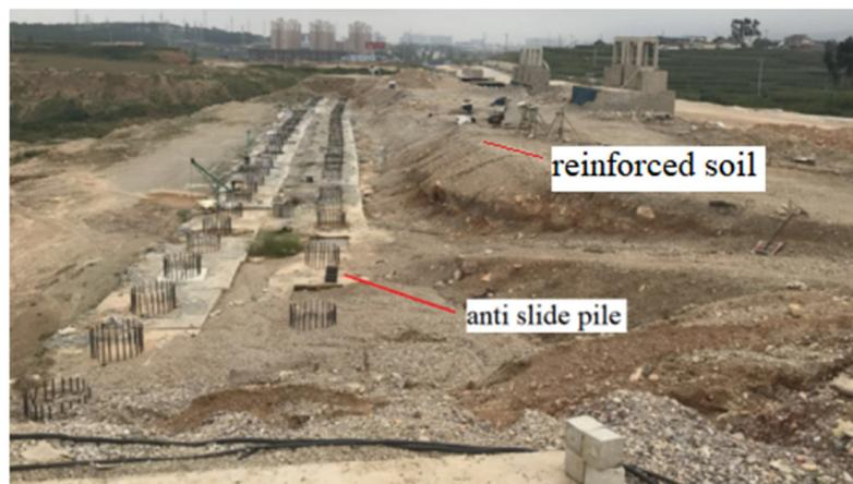
Figure 16. Site construction of reinforcement scheme.
