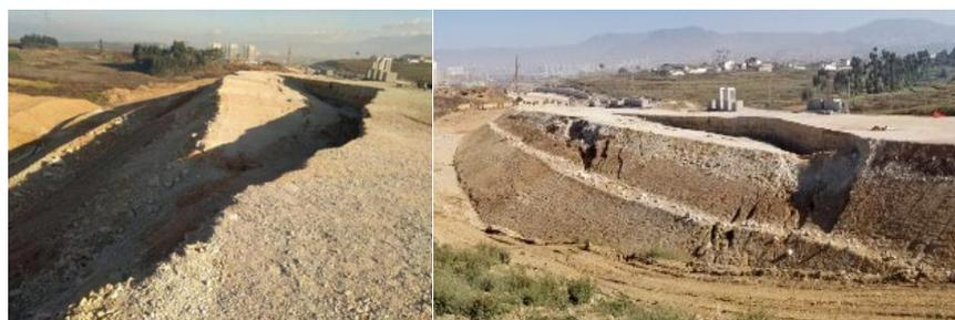
**Figure 12.** Tensile Cracks at the rear edge of Embankment Landslide.
