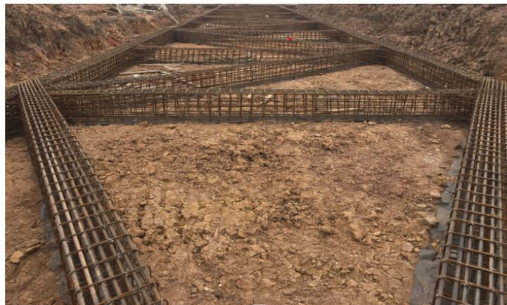
**Figure 3.** Steel bar binding of the inner brace.
