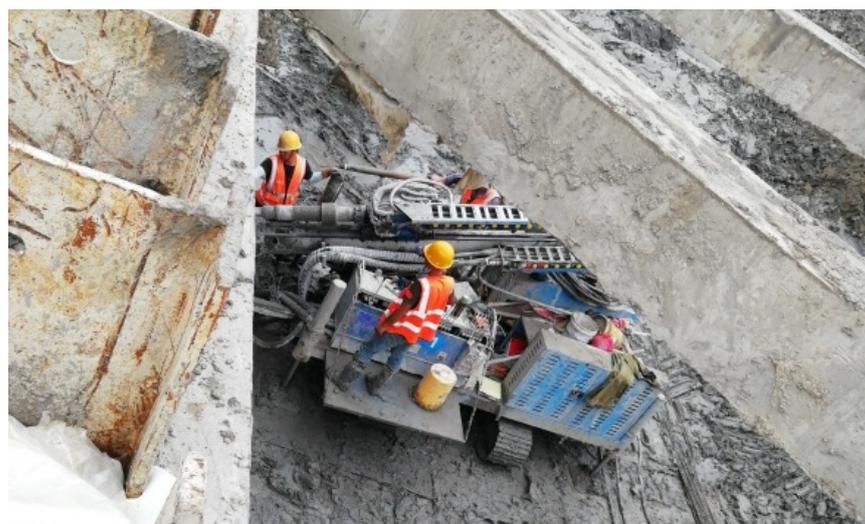
**Figure 6.** Grouting of anchor cables.
