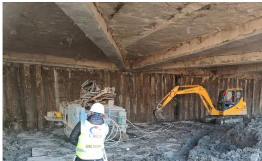
**Figure 5.** Drilling of the anchor cables.
