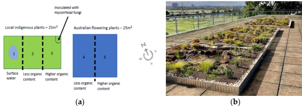
Figure 1. Details of green roof plots on Building M at Victoria University's Footscray Park Campus: (a) Green roof design, (b) Actual constructed green roof.
