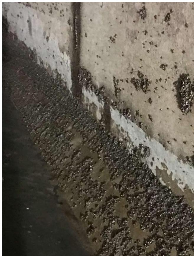
Figure 7. Freshwater mussels on an inverted siphon.
