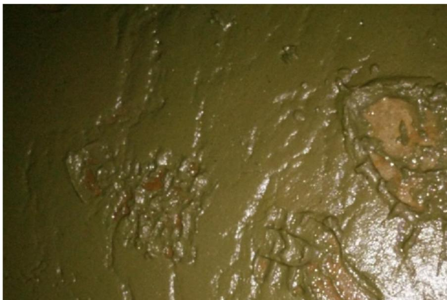
**Figure 8.** Sediments in an inverted siphon.
