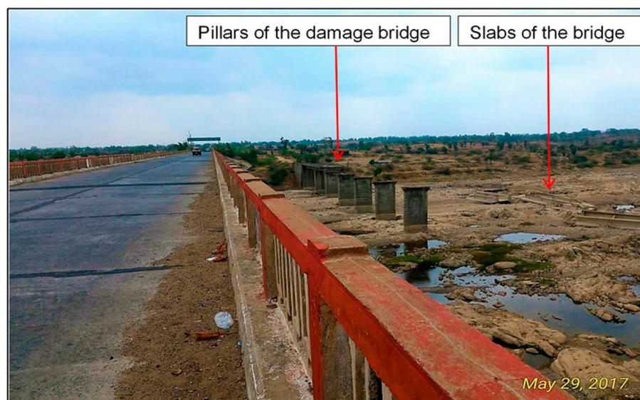
Figure 11. A view of collapsed Mahi Bridge as a result of the flood on 8 September 1973 from the new bridge on the Banswara–Sagwara highway near Kailashpuri (Sagwara, Rajasthan—captured by Hire, P.).
