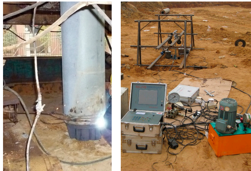
Figure 2. Welding and testing of O-cell.
