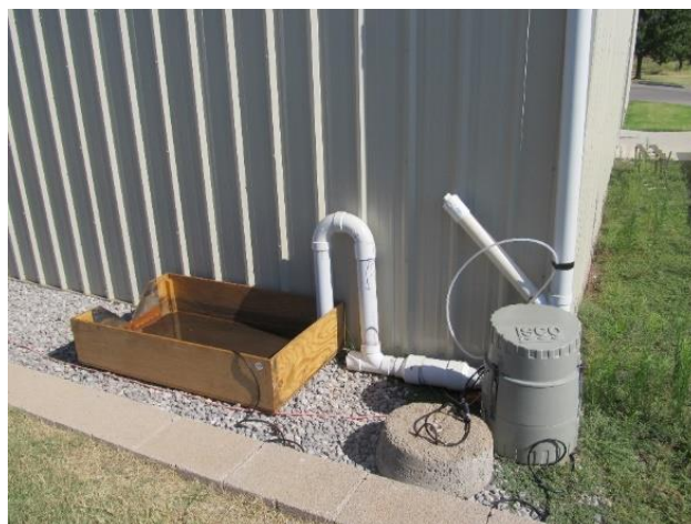
Figure 4. Example of the modified downspout and field sampling arrangement at the metal roof.
