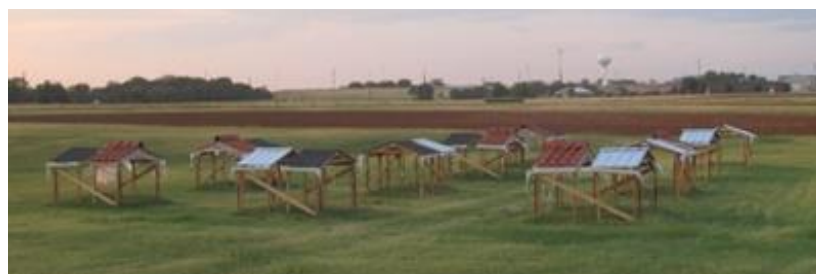
Figure 1. Eighteen constructed roof structures representing metal, asphalt shingle, and clay tile roofing materials used in the simulated rainfall events study.
