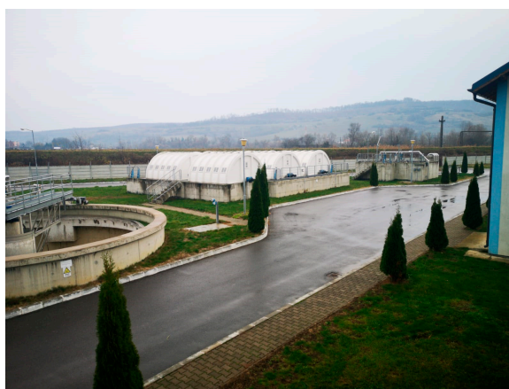
Figure 1. Dumbrăveni Wastewater Treatment Plant.
