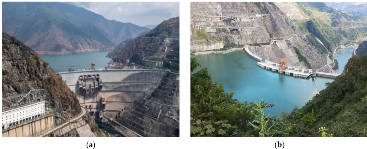
Figure 3. Aerial view of the dam. (a) Downstream view; (b) Upstream view.
