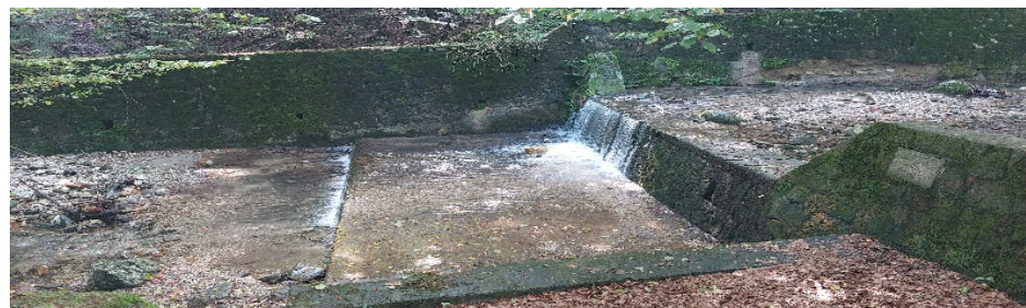
Figure 14. Example of a proposed bottom sill. Photo source: Author.
