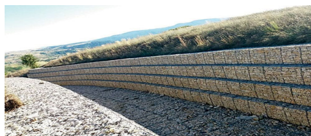
Figure 16. Example of a gabion wall proposed. Photo source: https://www.revistaconstructiilor.eu/ .
