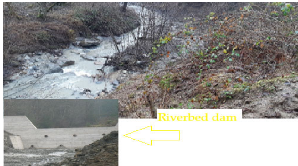
Figure 13. Proposed area for the construction of a riverbed dam and traverse anti-erosion stone dams. Photo source: author.
