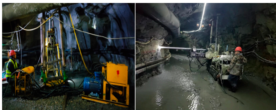
Figure 1. Site photographs of the horizontal grout curtain construction at the Cuihongshan iron–polymetallic mine.
