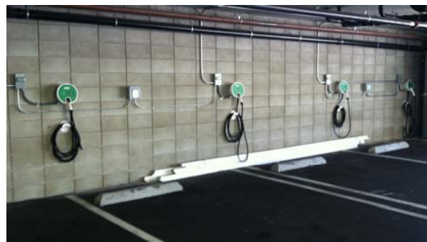
Figure 4: Multi-Unit Dwelling EVSE Installation
