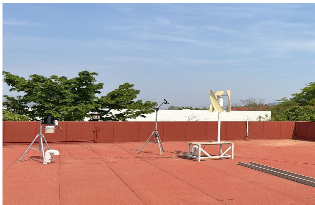
Figure 6. Wind Turbine Installation at the University of the Isthmus.
