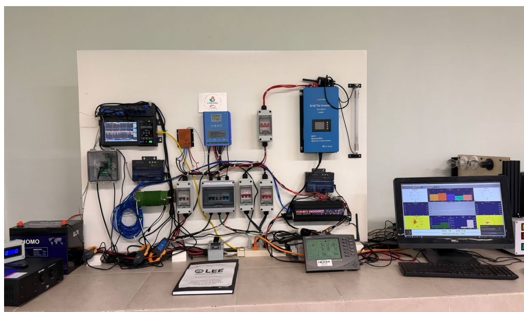
Figure 7. Experimental Bench and SCADA System.
