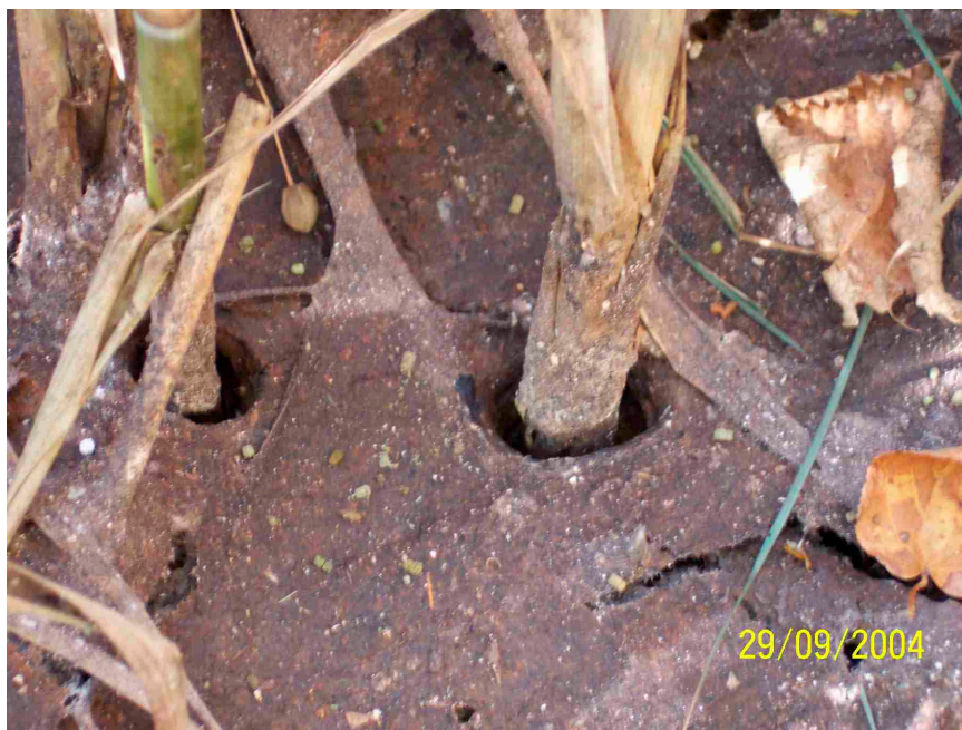
Figure 4. Openings in the sludge around the stems of Phragmites australis caused by the movements of the plants in the wind. These openings are important for maintaining a high water permeability in the sludge layer accumulated on the surface of the bed (photo: H. Brix).
