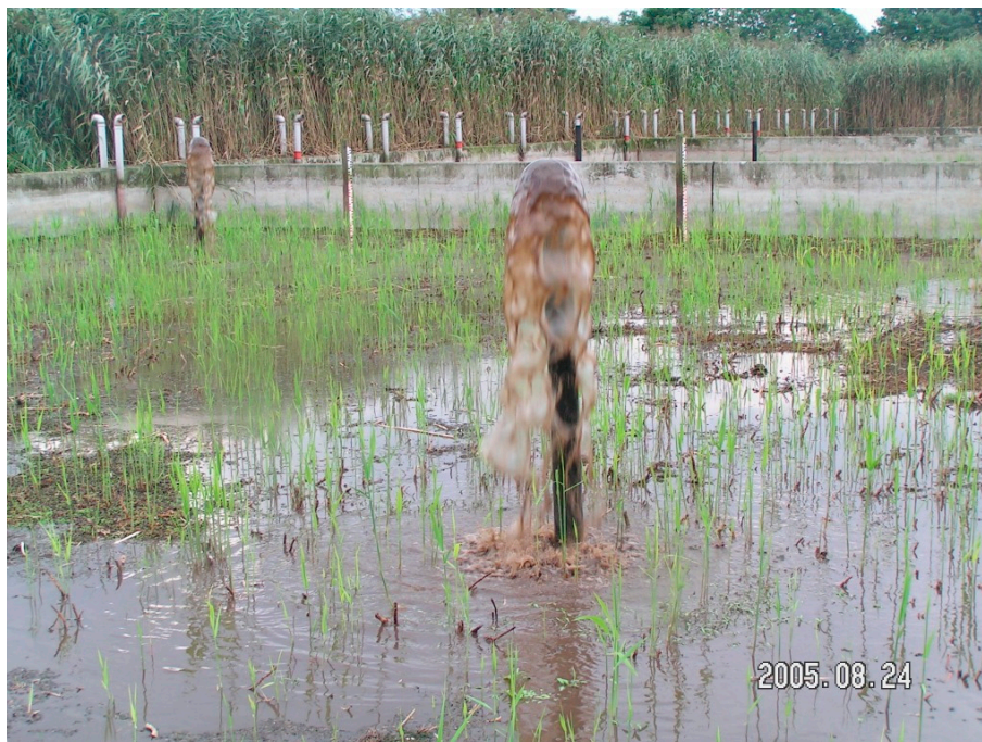
Figure 2. Vertical standpipes through which the liquid sludge is distributed over the entire surface of the bed. The picture shows a situation where a planted reed bed, after emptying, are being loaded again, and plants are regenerating from the rhizomes remaining in the growth layer (Photo: H. Brix).
