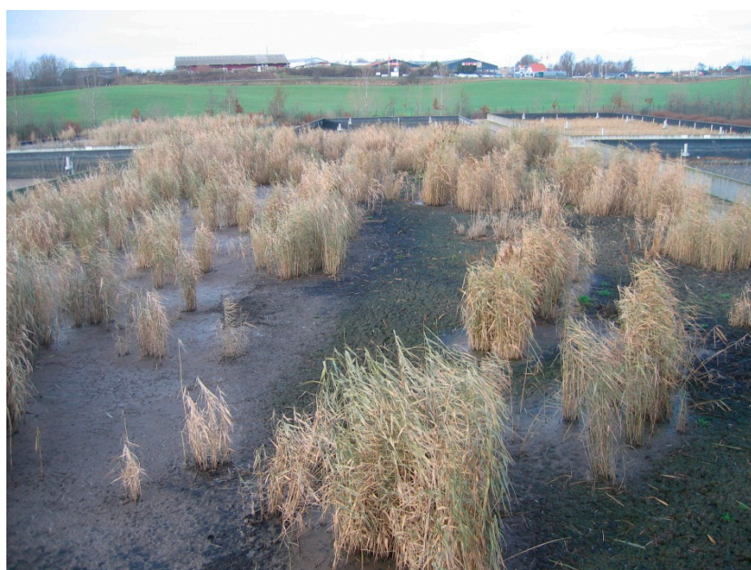
Figure 5. Typical sludge treatment reed beds with operational problems as indicated by the reduced and clumped growth of the reeds (photo: H. Brix).
