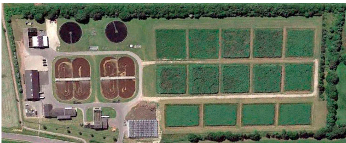
Figure 3. Overview of a typical 40,000 person equivalent sludge treatment reed bed system in Helsingør, Denmark (56°00'41" N; 12°11'29.4 E, February 2015). The surplus sludge from the activated sludge treatment systems to the left is pumped to fourteen reed beds in sequence. The water draining from the reed beds (reject water) is returned to the activated sludge tanks. When the beds are filled up with sludge after 8 to 12 years, the dewatered and partly mineralized sludge are used as a fertilizer in agriculture. The Helsingør system was established in 1996 with ten beds. The system was expanded with four extra beds in 2013.
